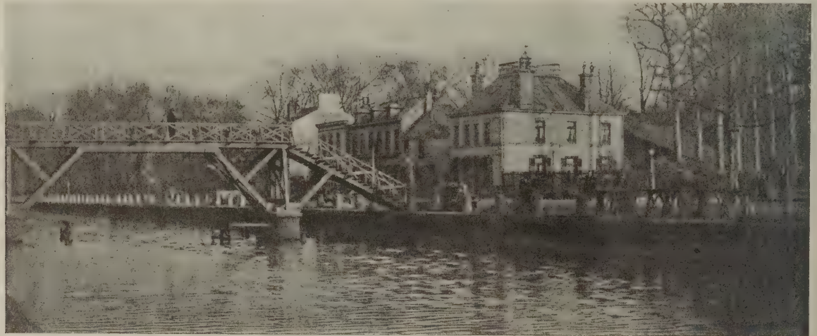
Until the Belgian Government is able to replace the beautiful stone bridges blown up by the Germans, temporary footbridges like those shown in the illustration will serve the needs of the people of Lillie. The reopening of the canal on which the city is situated, which was also wrecked by the retiring Teutons, has restored traffic through the inland waterways to pre-war normality.
